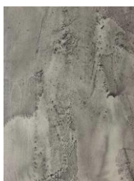
Concrete rough grey
